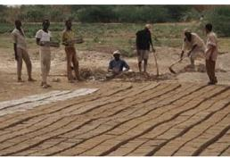
Figure 2: Slop-moulding and drying of bricks. Photo: Practical Action
